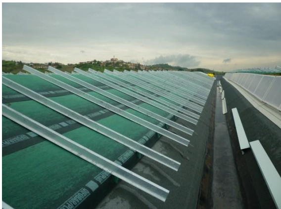
Placement of PV fastening outline
